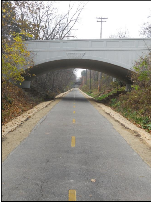
Image 1 (Steven Krueger, 11/2012) shows a typical span of a Madison bike path (Class I). This image shows a span of the Southwest Commuter path that passes under Spooner Street. It is important to note the attempts at the path to not only be functional but also to be aesthetically pleasing as seen by the style of the bridge.
