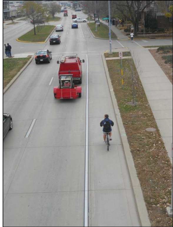
Image 8 (Steven Krueger, 11/2012) features a bike lane (class II) along a high volume street (Park Street). The lane is separated only by a painted line.
