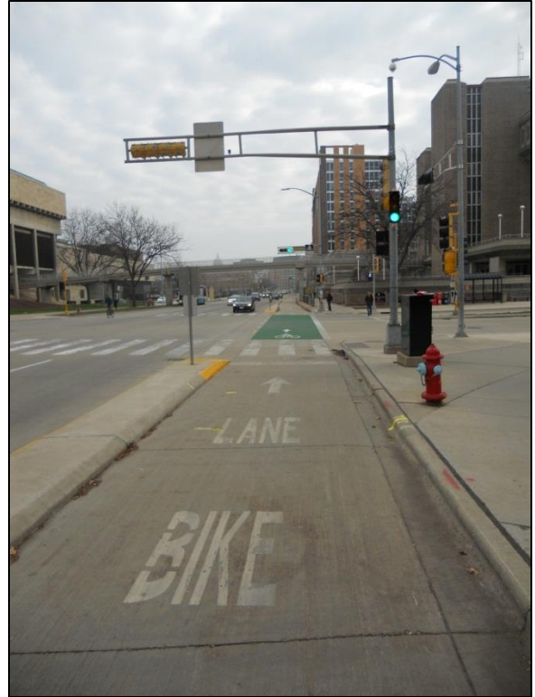
Image 5 (Steven Krueger, 11/2012) is the bicycle path (class I) traveling east down University Ave. The path travels against traffic and is separated by a raised divider. Notice the green path going through the intersection to reinforce separation of the lane from traffic.
