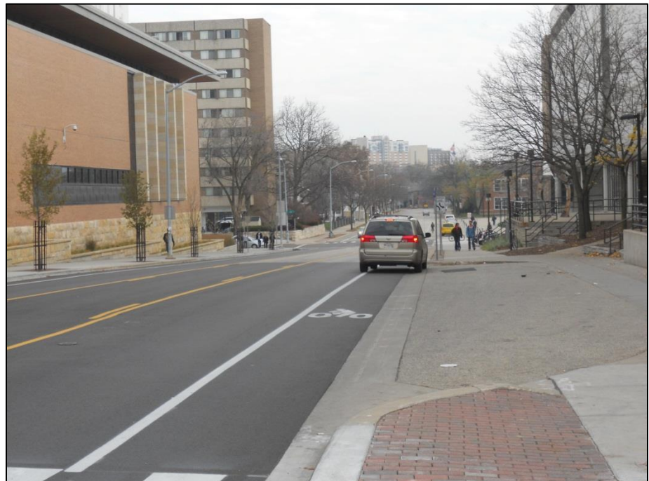
Image 12 (Steven Krueger, 11/2012) presents a common problem with bike lanes designated with painted lines (class II). A motorist has illegally parked in the lane restricting bicycle traffic and potentially putting bicycle riders at risk while attempting to overtake.
