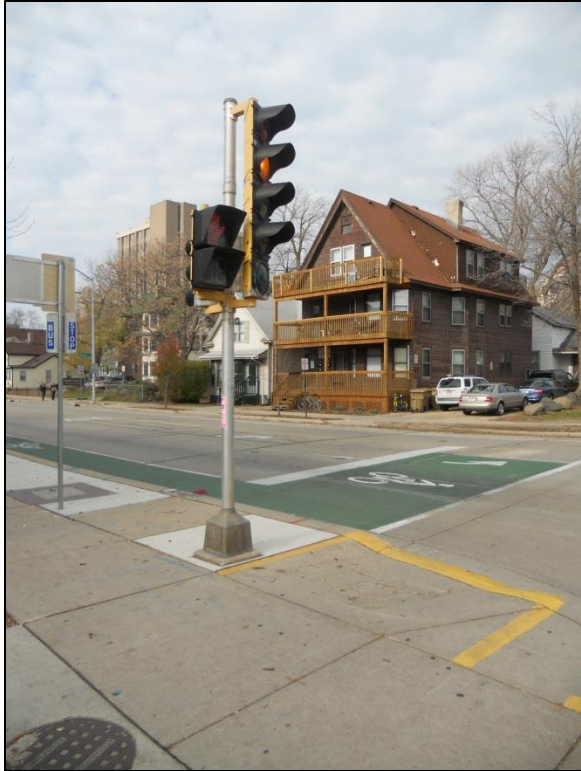
Image 7 (Steven Krueger, 11/2012) is an example of a combination green lane and bike box on street with a designated bike lane (Class II). Here bicycles stop in front of traffic in the designated green area. This creates a clear area designated for bicycles separated from the rest of traffic. It also allows for safer left turns for bicycles.
