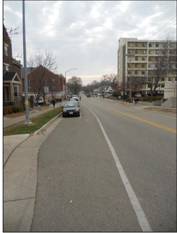
Image 2 (Steven Krueger, 11/2012) shows an example of a bike lane (class II). This image was taken on the intersection of the SW Commuter path and Dayton Street. A bike lane is a designated lane of a road restricted to bicycle use. It separates cyclists and motorists by a painted line, raised divider, or curb. This lane is separated by a painted line and is situated between a parking and driving lane.
